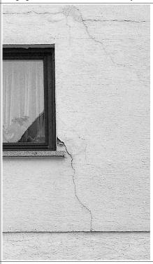
**Pre-Treatment:** Widen the structural crack approx. 1 cm wide and 1 cm deep (U-shaped) and remove dust. Prime liberally with Dupa-grund to the saturation point.
